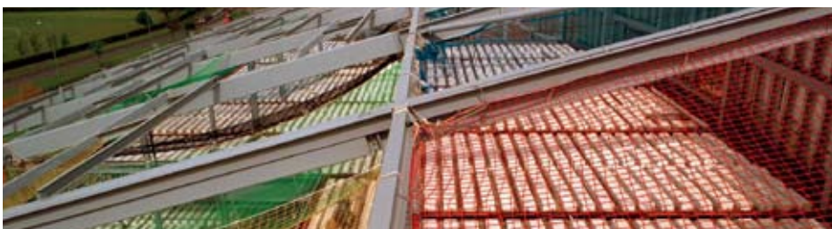
Figure 1.10 Safety netting is used when working at the highest point
