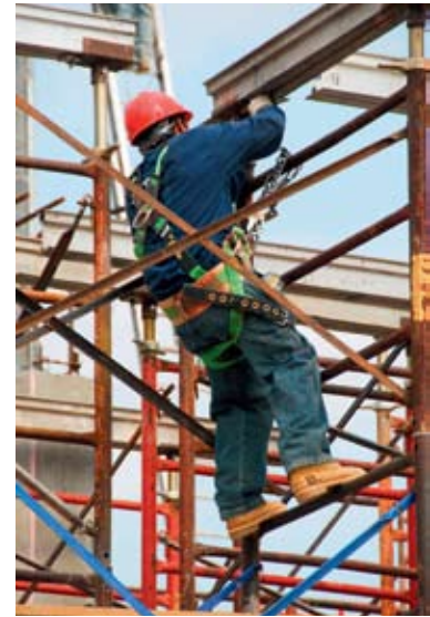
Figure 1.9 A harness and lanyard can prevent a worker from falling to the ground
